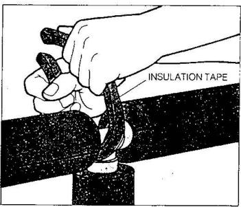
2 Taping the fittings. Cover the pipe fittings with insulation tape ¼ inch thick. Be sure to cover the fittings completely: no part should be exposed to air. To complete the job, wrap both the pipe and the fittings in aluminum foil.
